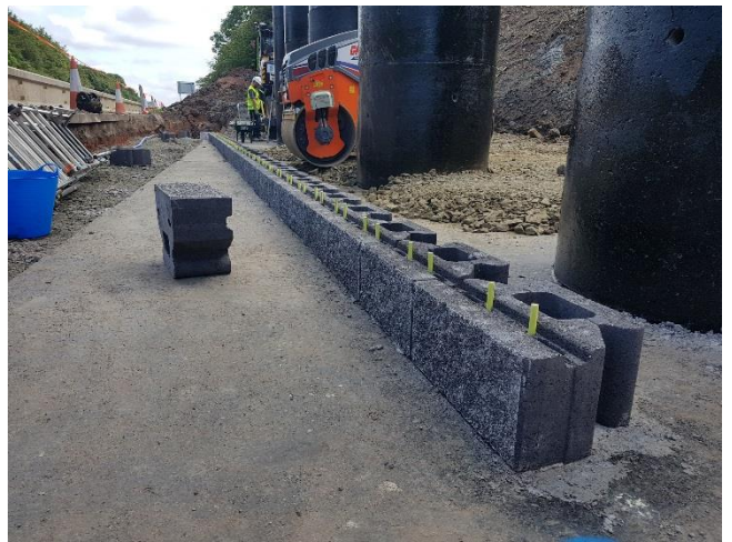
Reinforced soil facing blocks with waterproofed manhole sleeves behind
