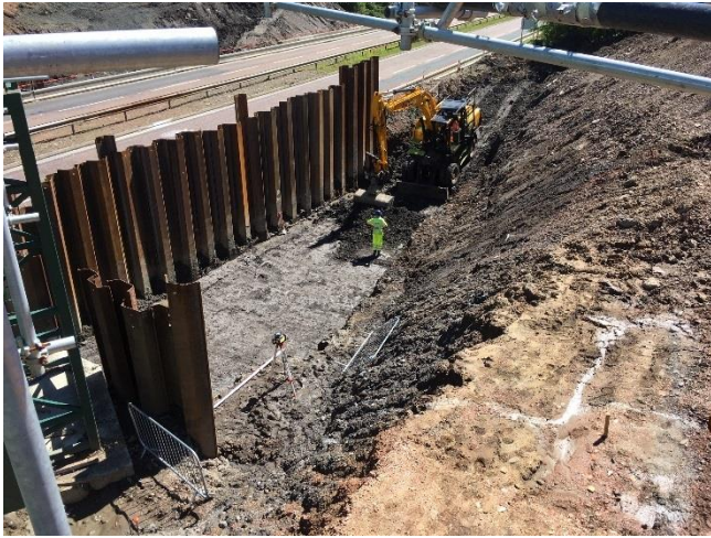
West - Placement of structural fill below foundations
