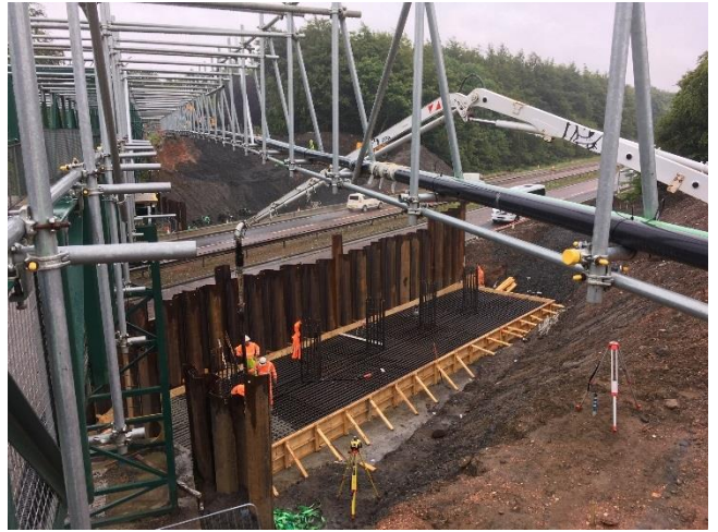
West - Installation of steel reinforcement
