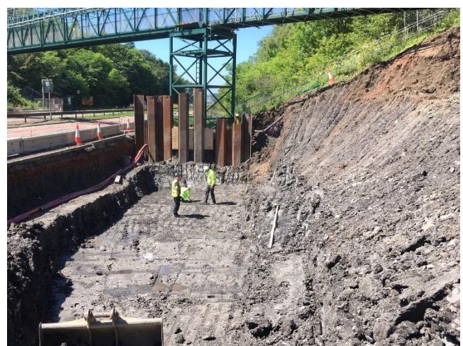
East - Inspection of sub-formation clay
