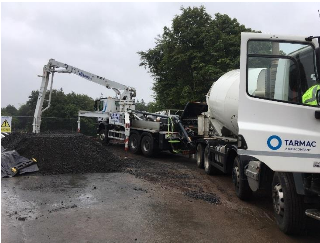
West – Concrete delivery and pumping
