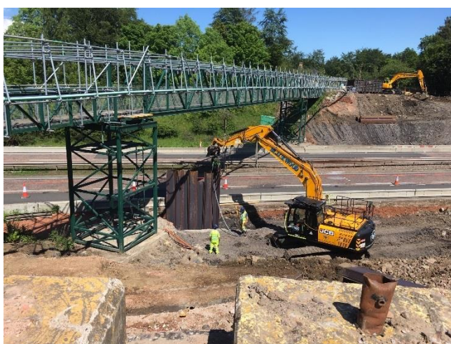
West - Installation of temporary sheet piles to support A90
