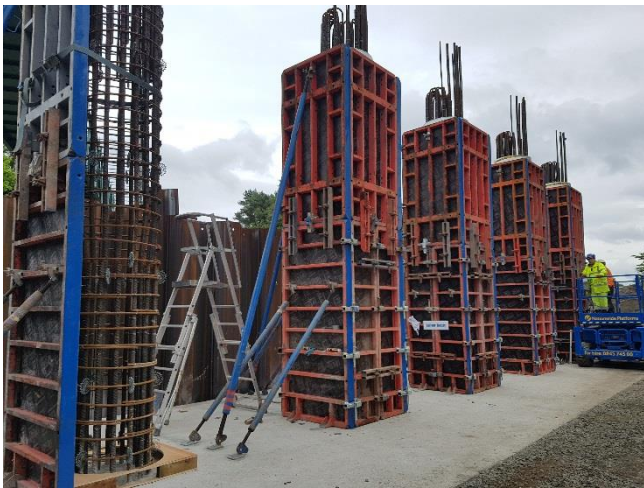
West columns prior to pouring
